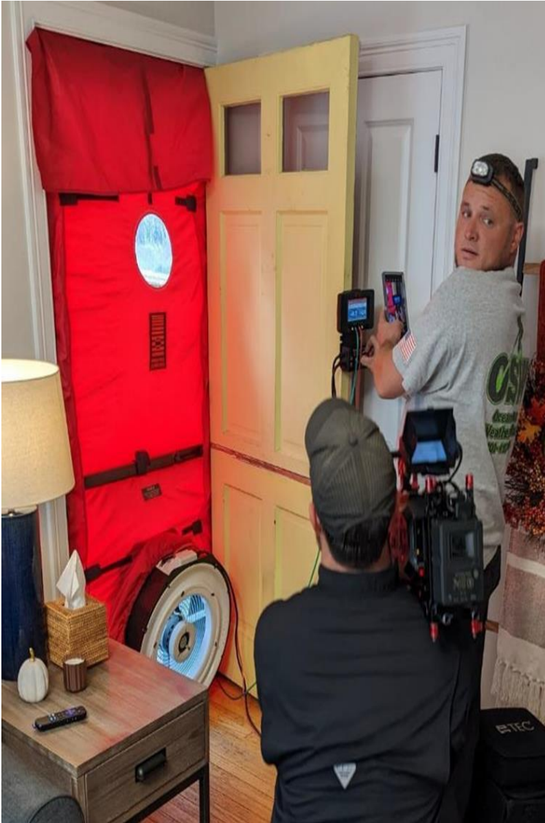
Home Energy Assessment Blower Door Test
